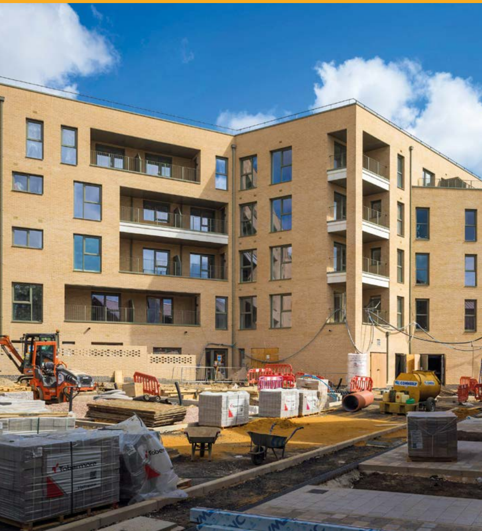
Coppice Wood Lodge construction
